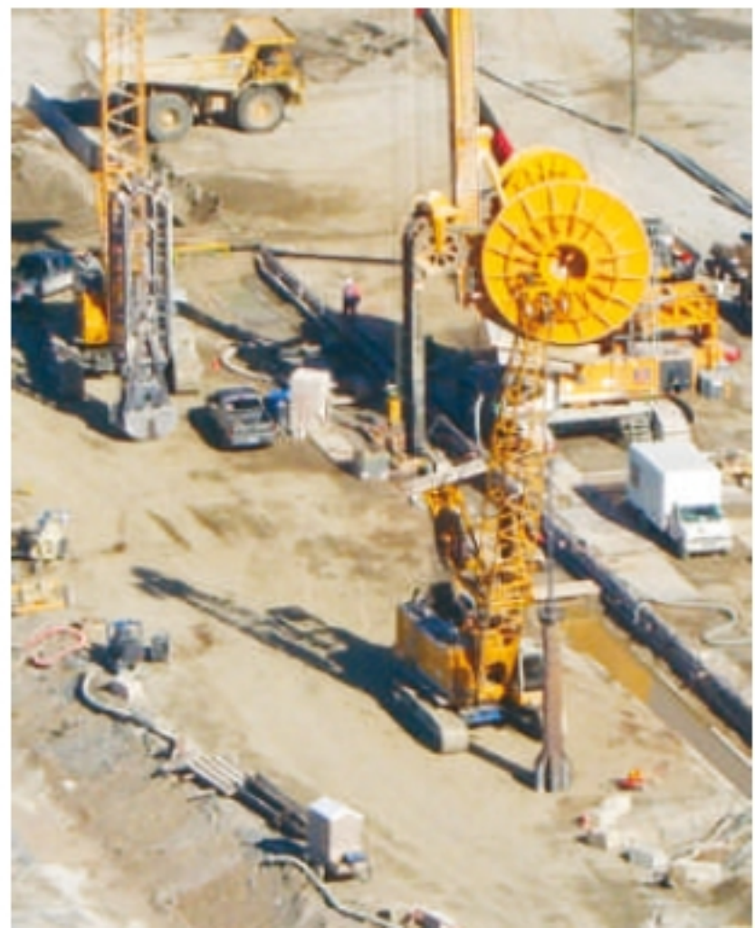
Cut-off wall in progress
